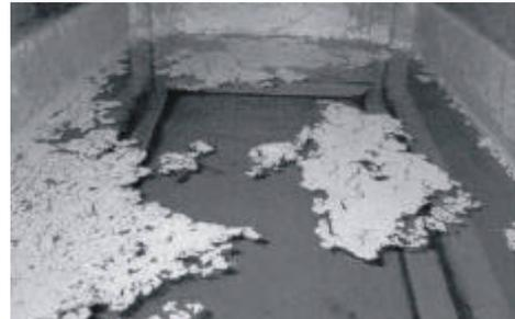
Should any significant level of debris be observed internally and / or water quality is less than the wholesome level required it is recommended the vessel be drained, internal surfaces washed down, the tank re-sterilised and the water quality rechecked before returning it to service.
